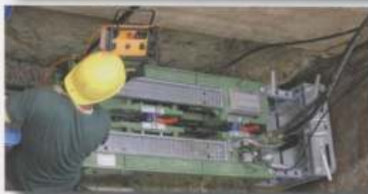
Above and left: Long pipe bursting from pit to pit
