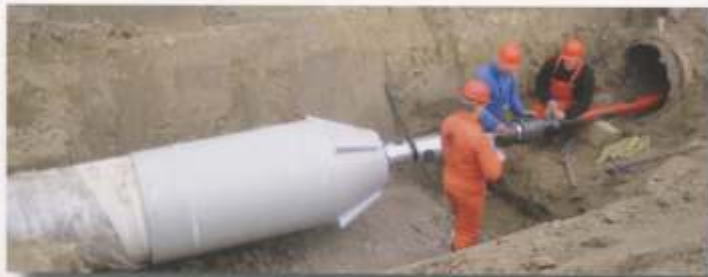
Above and left: Long pipe bursting from pit to pit
