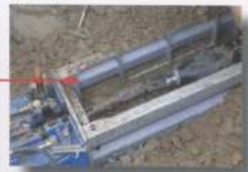
New pipe in the target pit
