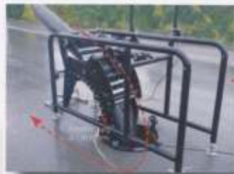
Long pipe installation through a manhole using BURSTFORM.
