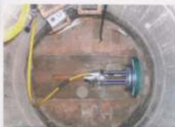
Stable connection of short pipes using BURSTFIX
