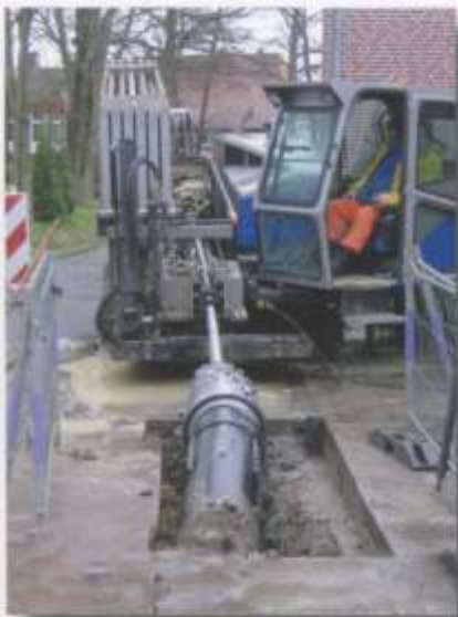
Bore head with sonde
