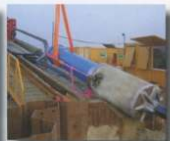
HDD-Assist application: Loosening of stuck drill rods
