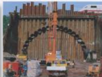
Construction of a pipe roof
