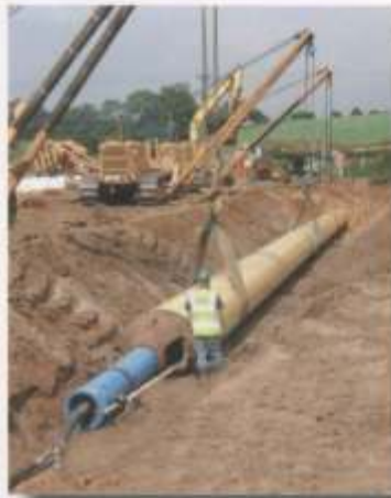
... in pipeline construction
